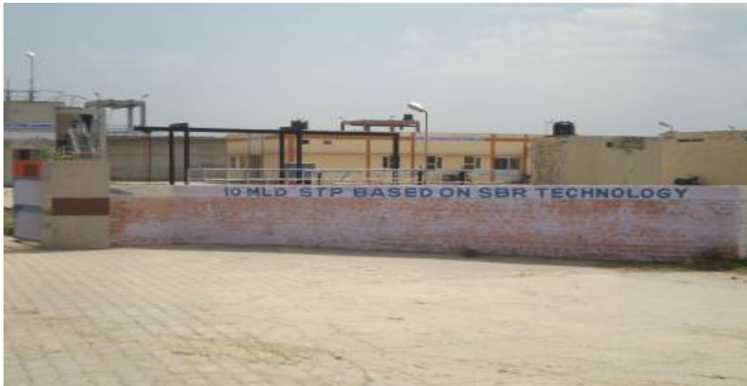
Figure 1: 10 MLD, STP at Kaithal town (Haryana) India.
